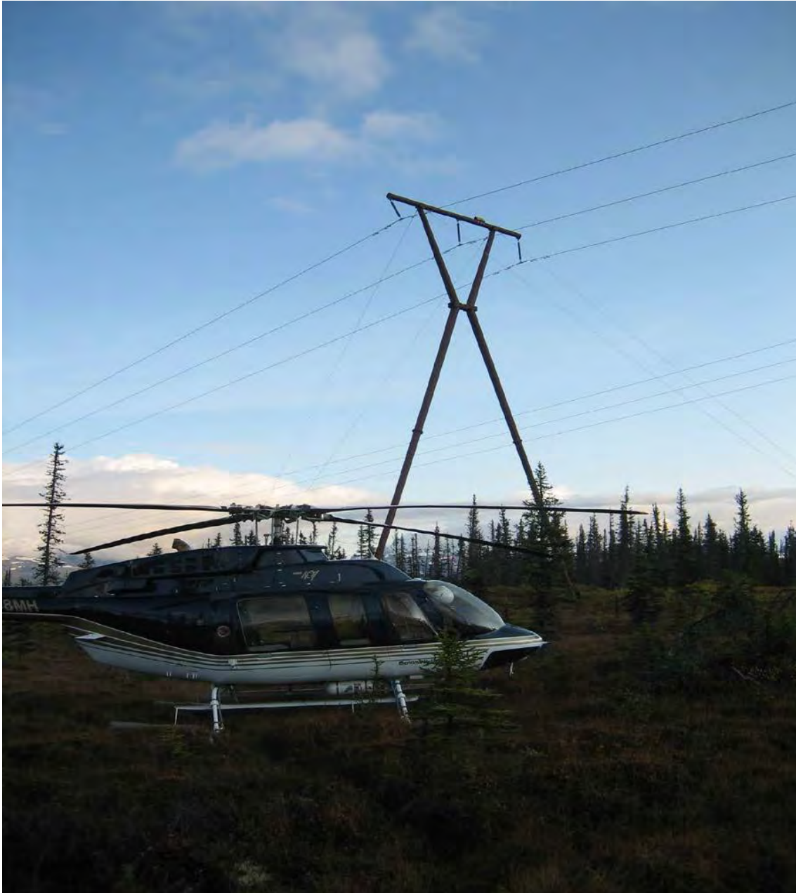
HEA Line Inspection Project
